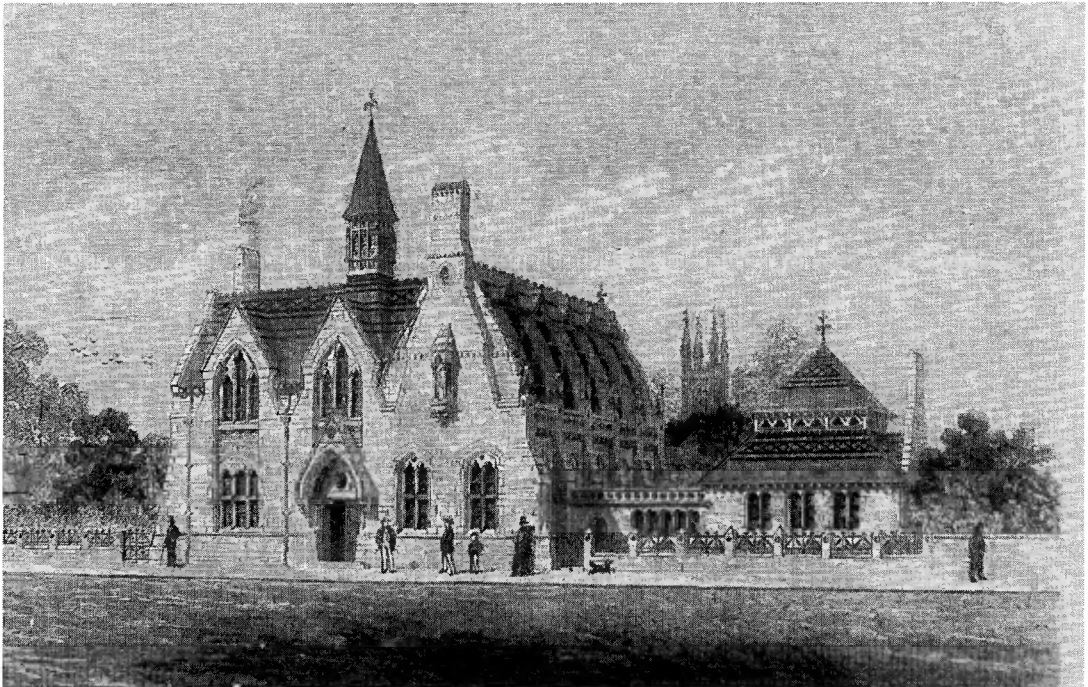
Fig. 2. Gloucester Schools of Science and Art, Brunswick Road: design for the original building ( The Builder , 17 June 1871). The museum was on the left of the entrance and the art school above, with its tall north lights on the right overlooking the chemical laboratory.
