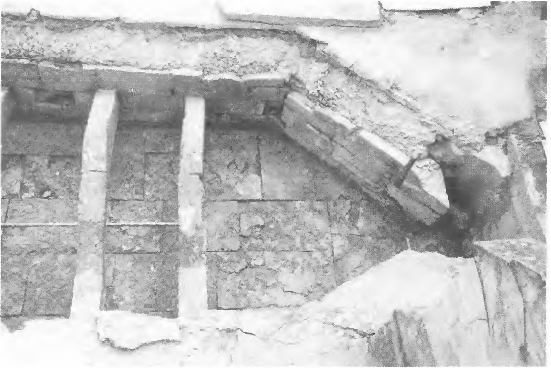
Fig. 5. View of the west end of the tank showing the funnel sluice and concrete 'shaft'.
