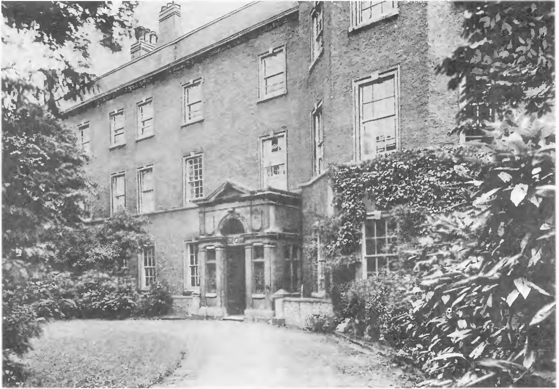
Fig. 2. A view c. 1920 of the front (northern) elevation of Redland Hill House before demolition of the western half (Bristol Central Reference Library B21205: reproduced by kind permission of the library).
