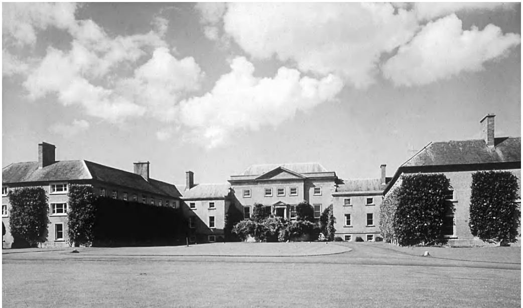
Fig. 2. Earnshill (copyright: Country Life Picture Library). The central Palladian block attributed to Colen Campbell is flanked by the two massive wings built post-1758.
