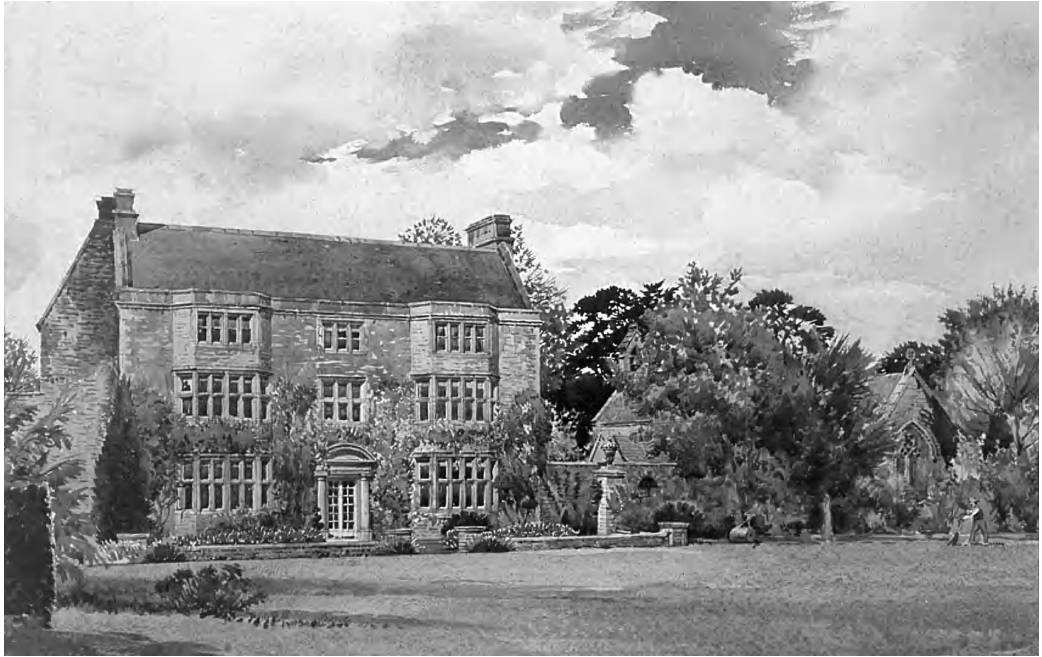
Fig. 1. The Manor House, Burnett: from a watercolour by A.C. Fare, R.W.A.. The 17th-century (Whitson) part is on the north (right hand) side: the 18th-century section to the south of the Georgian doorcase has fenestration re-used from parts of the 17th-century building then demolished.
