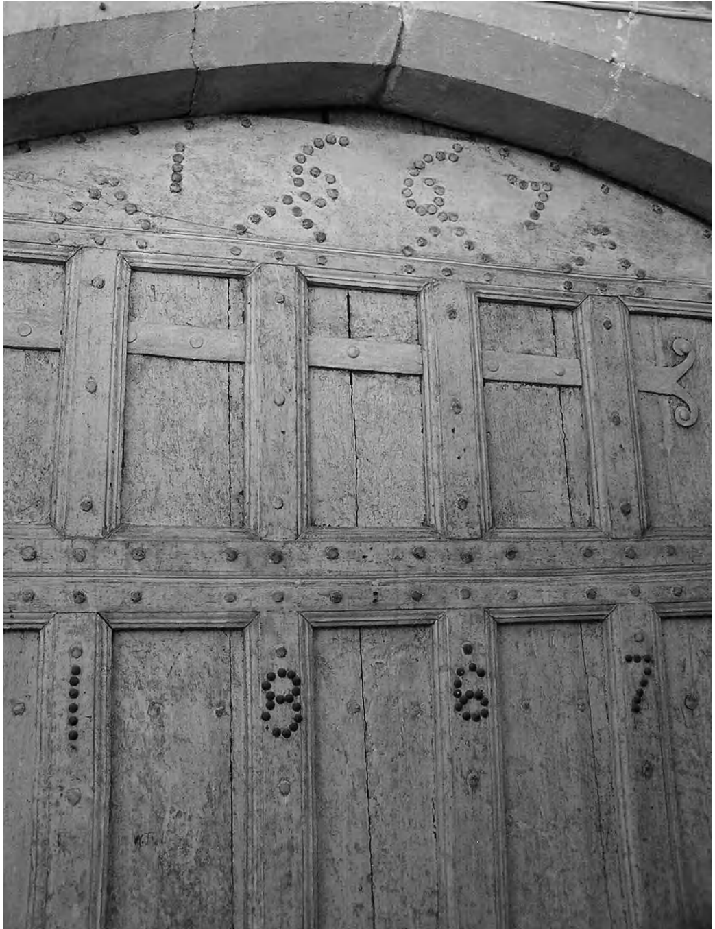
Fig. 3. The door leading to the consistory court dates from soon after the foundation of the abbey in 1140. The cladding was affixed to the door and the date 1667 marked with nails at the top of it when the court room was refurbished by the registrar, Edward Pownall. Photograph by Philippa Johnson.
