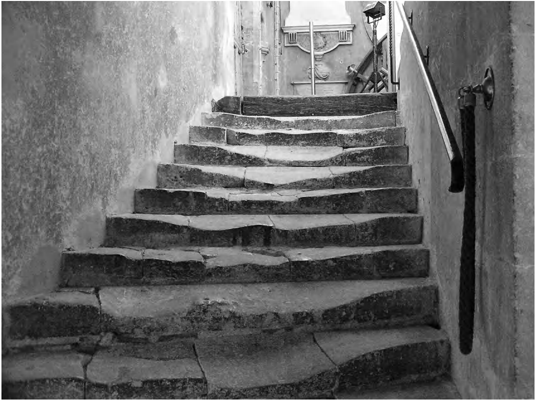
Fig. 1. The former night stairs of the Augustinian abbey, now badly worn by the feet of those attending the Bristol consistory court. Photograph by Philippa Johnson.
