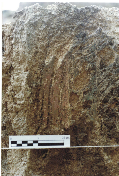
Fig. 6A. (right) Photograph enlarged to show vestiges of paint on the wall-plaster in situ on the cellar's south wall.
