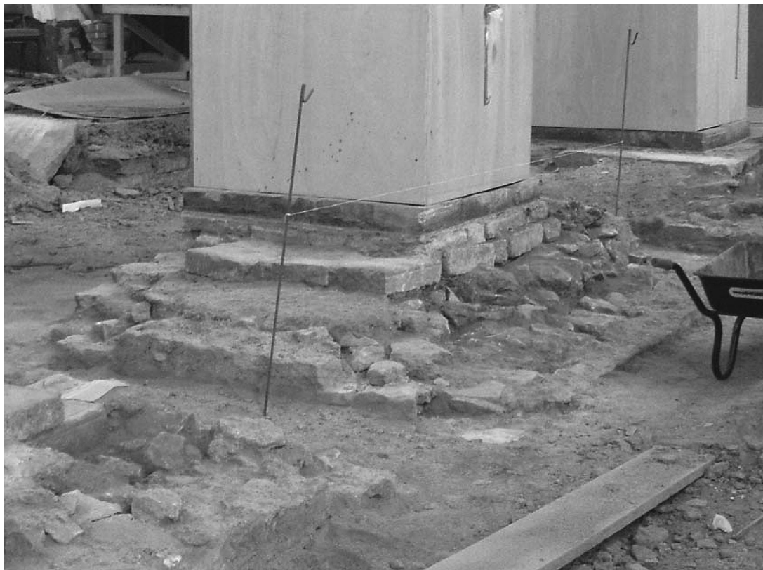
Fig. 10. The multi-period base of the central pier in the south nave arcade.
