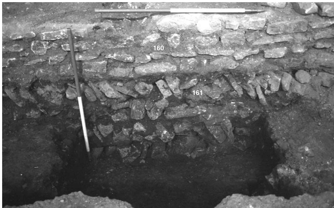
Fig. 5. The wall 160, and footings 161, under the south aisle wall.
