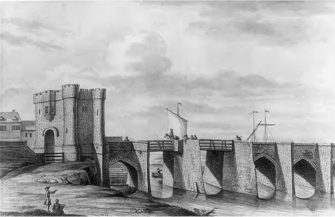
Fig. 2. Westgate Bridge from the north: pen and wash drawing by Bernard Lens (c.1681–1740). The waterwheel drove a pump from 1694 until the 1740s. By 1789 the second span from the gate had been rebuilt in masonry and the fourth had become a round, not a pointed arch. The fifth and sixth, which lay outside the river channel, were walled up before 1818. Copyright Gloucester City Museum and Art Gallery (cat. no. 1801).
