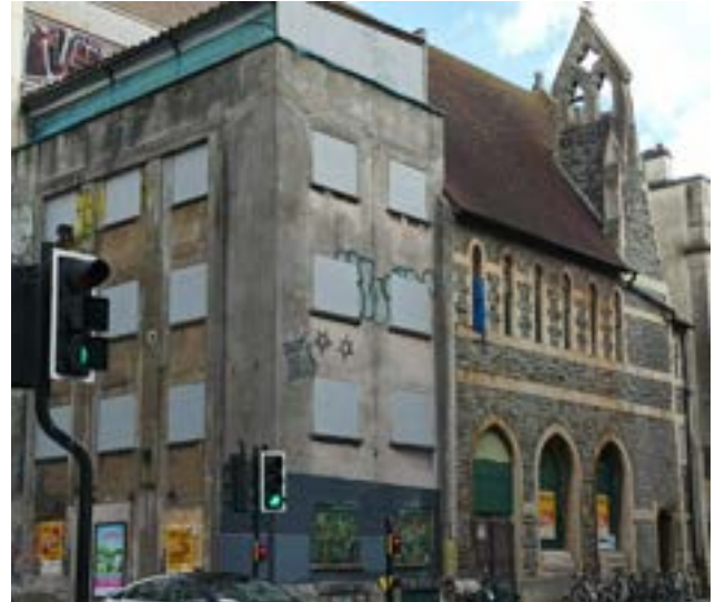
The former Seamen's Institute and chapel viewed from Prince Street.
